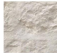
Lime plaster walls
