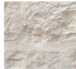
Lime plaster walls
